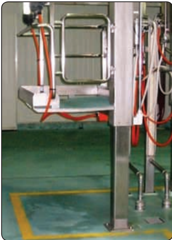
Lines mark restricted access areas underneath and around RFPs.
