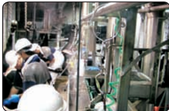
Example of fall restraint harness system to prevent the worker reaching the edge of the platform. Note the slide ring attachment which enables easy movement along the platform.
